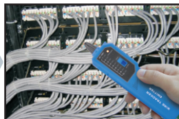
Trace cable at the other end with receiver
